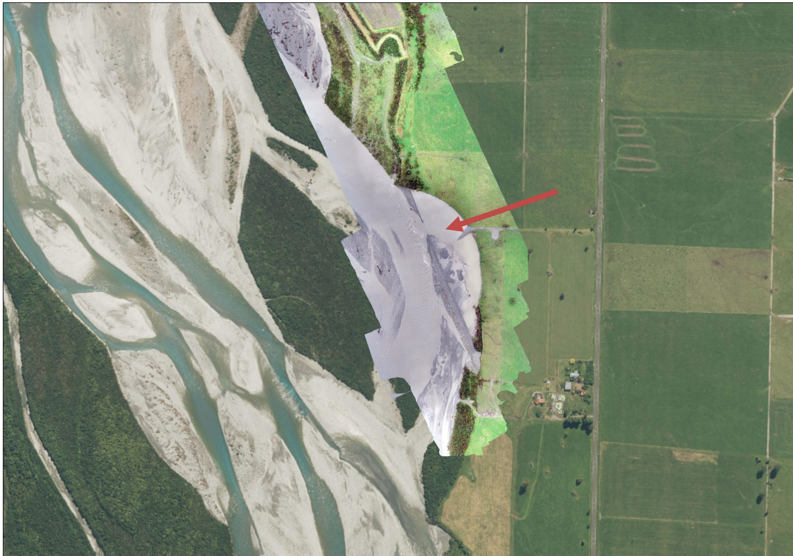
Photo 3: Wanganui showing breach at Raymonds bank
