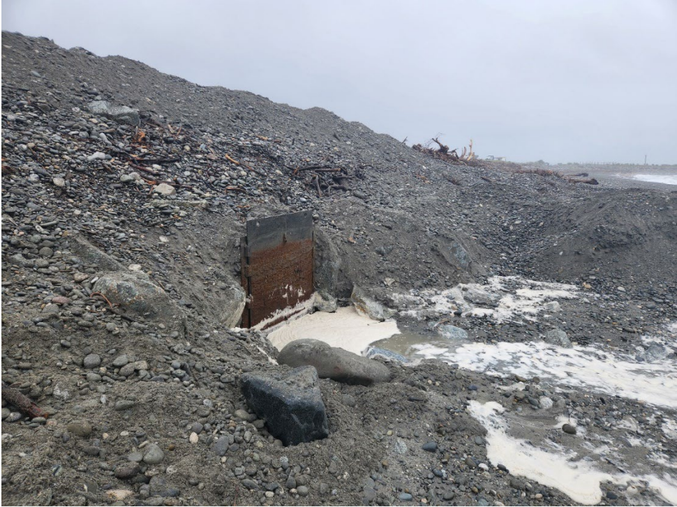
Photo 1: Slide gate uncovered
